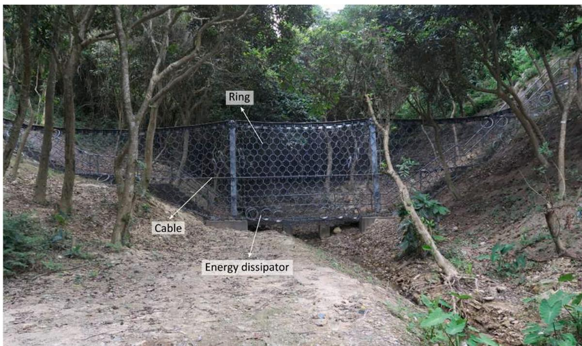
Fig. 1. A flexible ring net barrier for mitigation of debris flow in Hong Kong.
